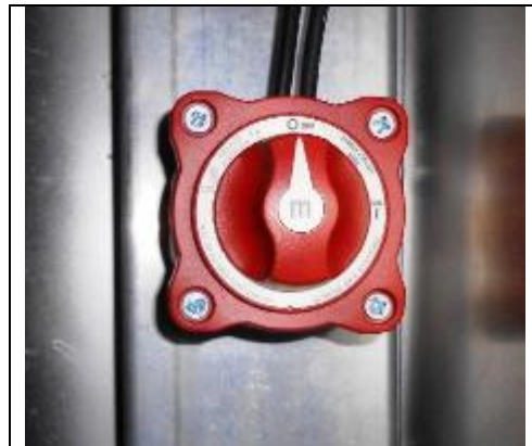
Figure 6-1 – 12 Volt Disconnect Switch
