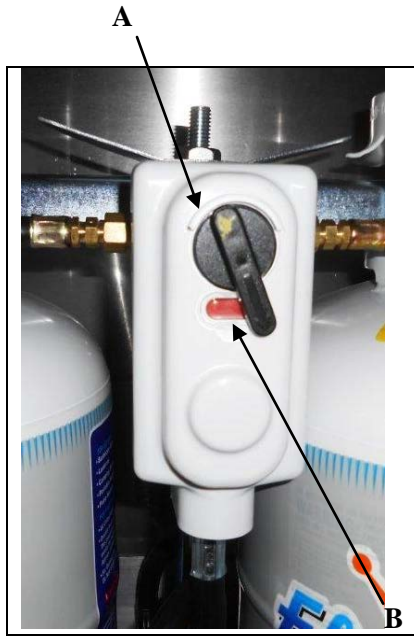
Figure 4-1 – LP Gas Regulator
