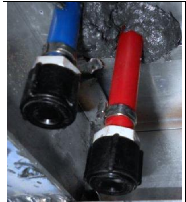
Figure 5-6a – Low Point Drain Lines
