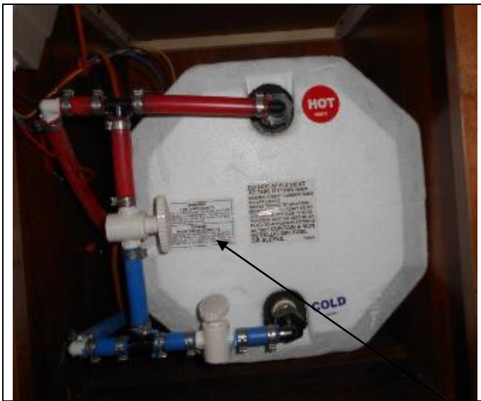
Figure 12-2 – Water Heater Bypass Valve
